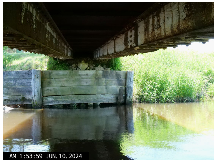
South Abutment & Retaining Wall
