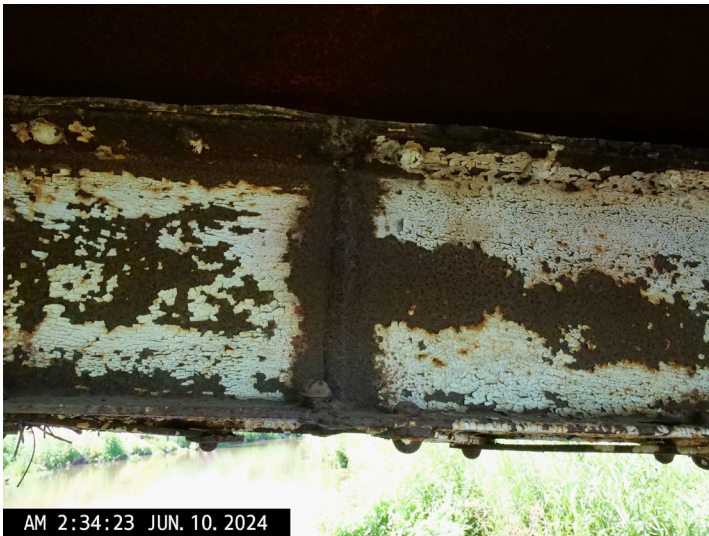
Girder Welded Spice
