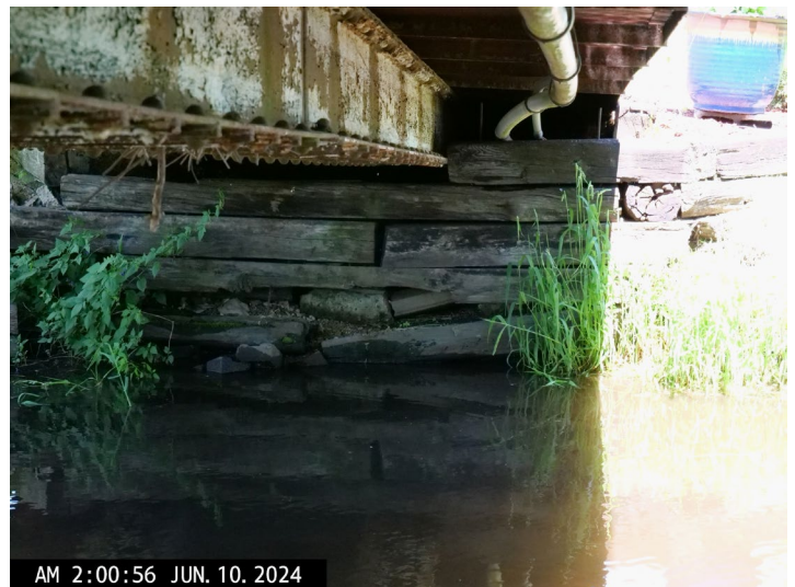
North Abutment Retaining Wall
