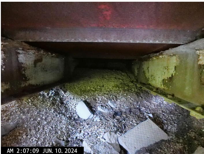
North Abutment Close Up
