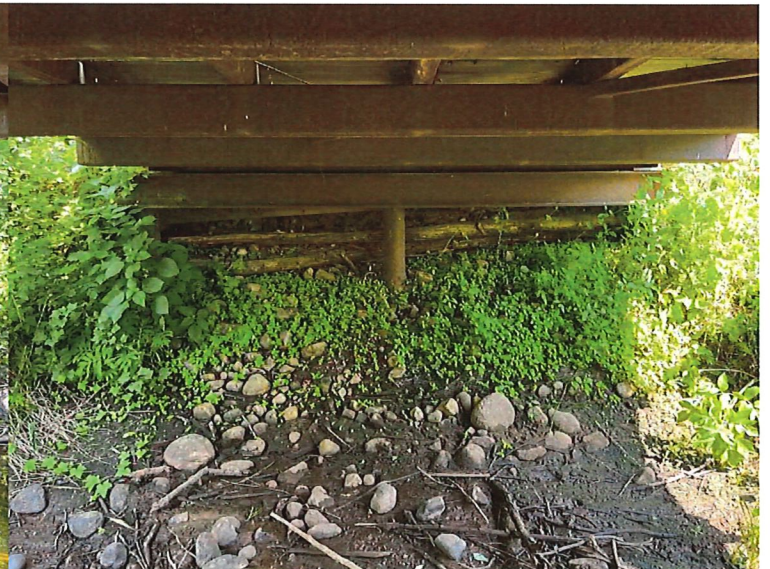
Bridge Substructure and Abutment Looking East
