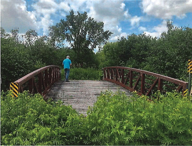
Bridge Deck Looking West
