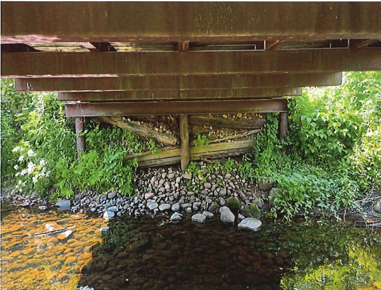
Bridge Substructure and Abutment Looking West
