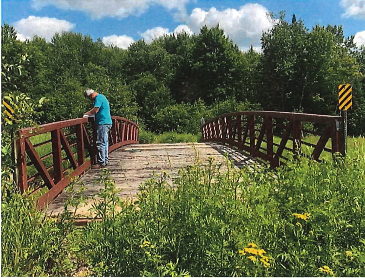
Bridge Deck Looking West
