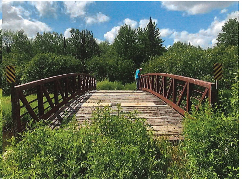
Bridge Deck Looking East
