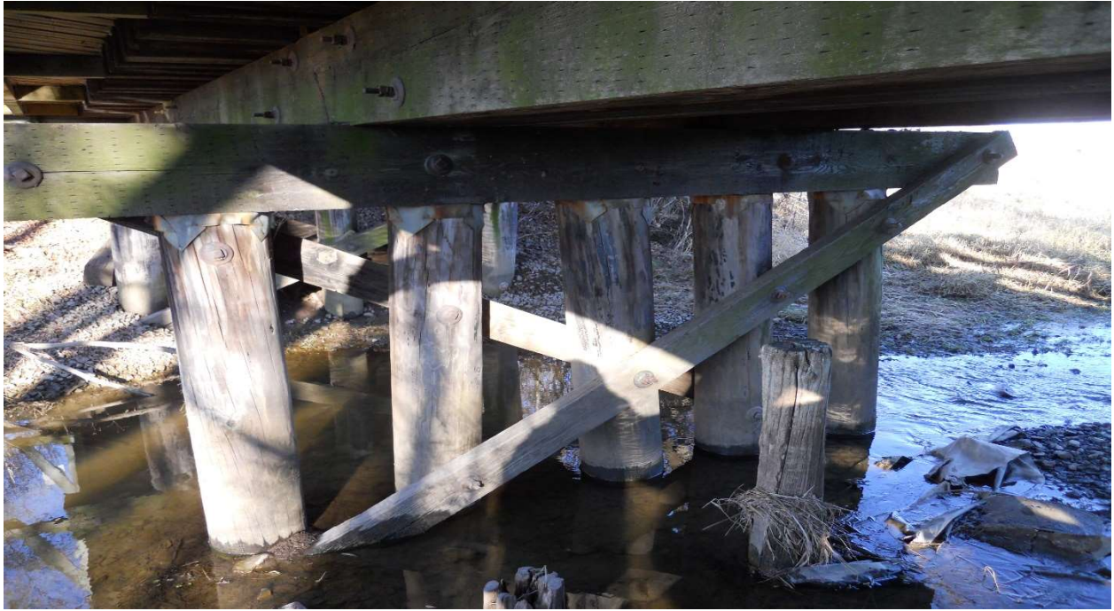
Typical pier, looking northwest.
