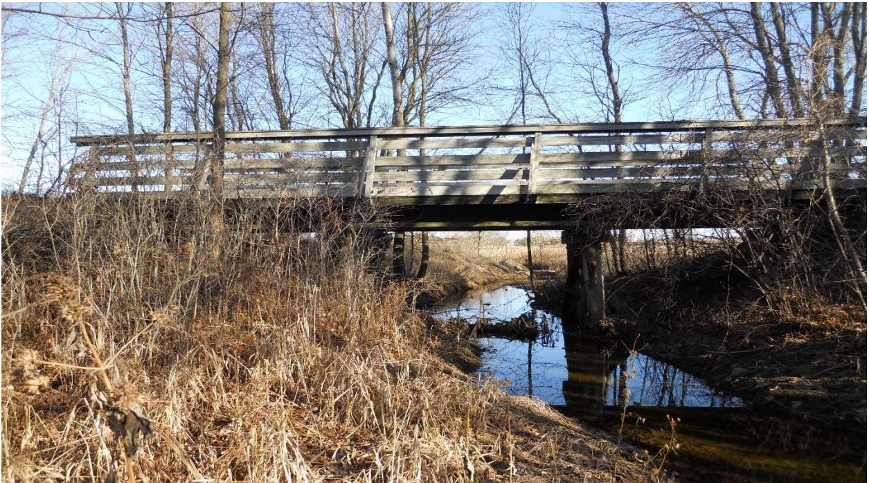
South fascia, looking north.
