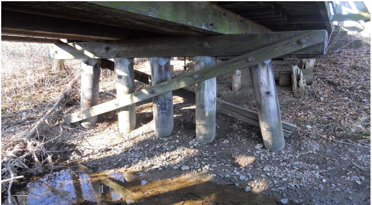
Typical pier, looking southwest.
