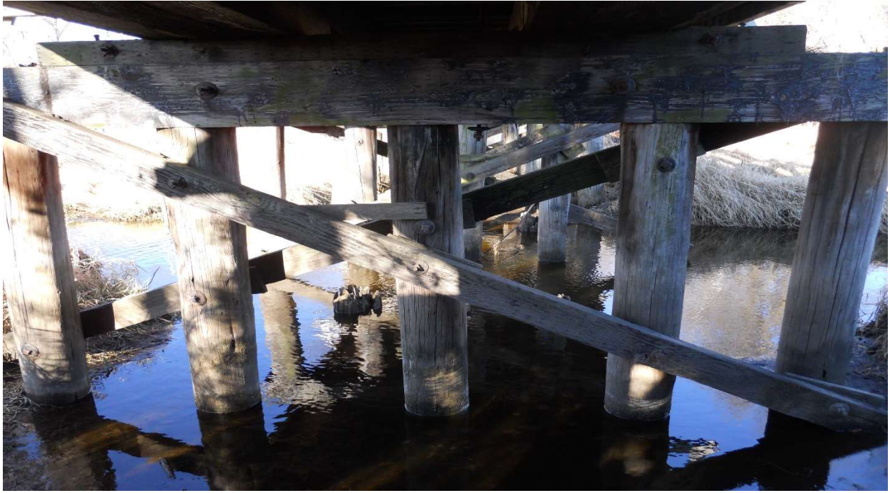
Typical pier, looking west.
