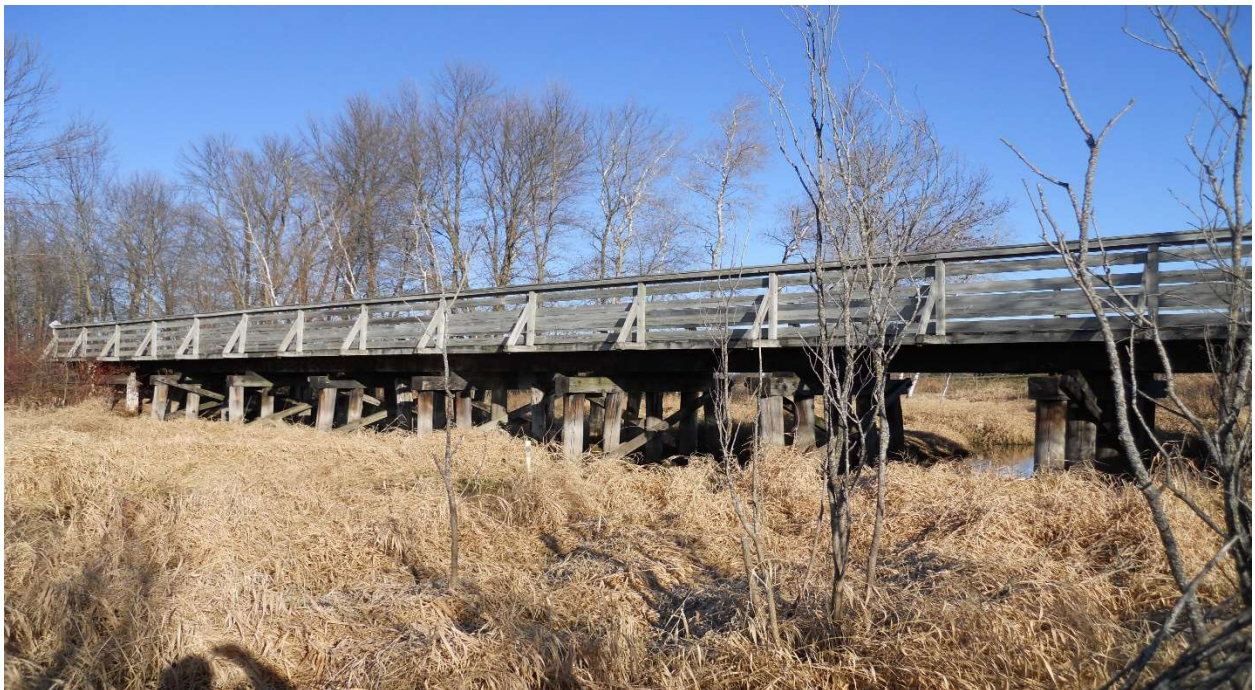
South fascia, looking northwest.
