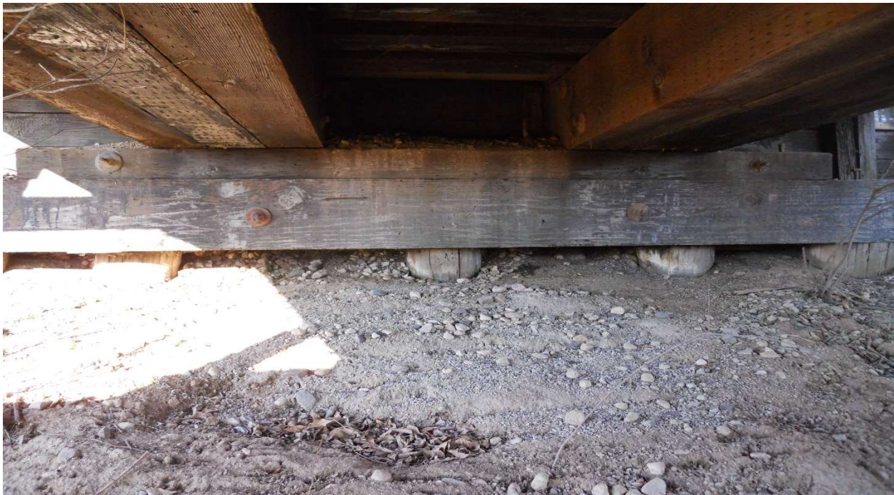
West abutment, looking west.
