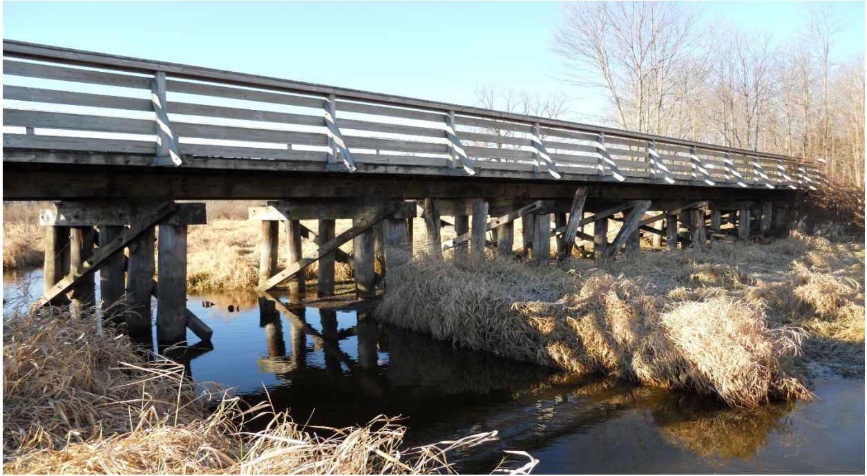
North fascia, looking southwest.
