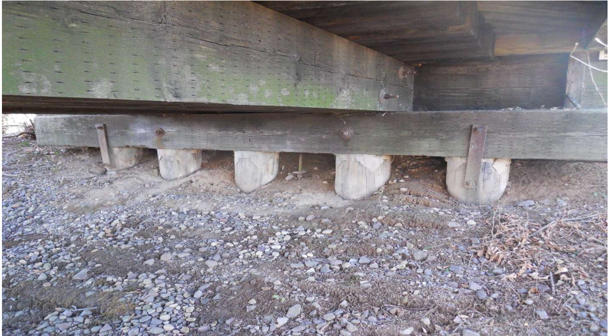
East abutment, looking northeast.
