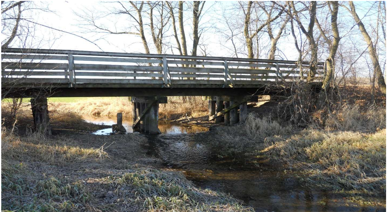
North fascia, looking southwest.
