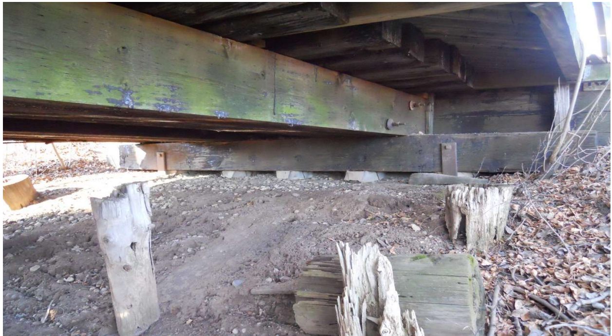
East abutment, looking southeast.
