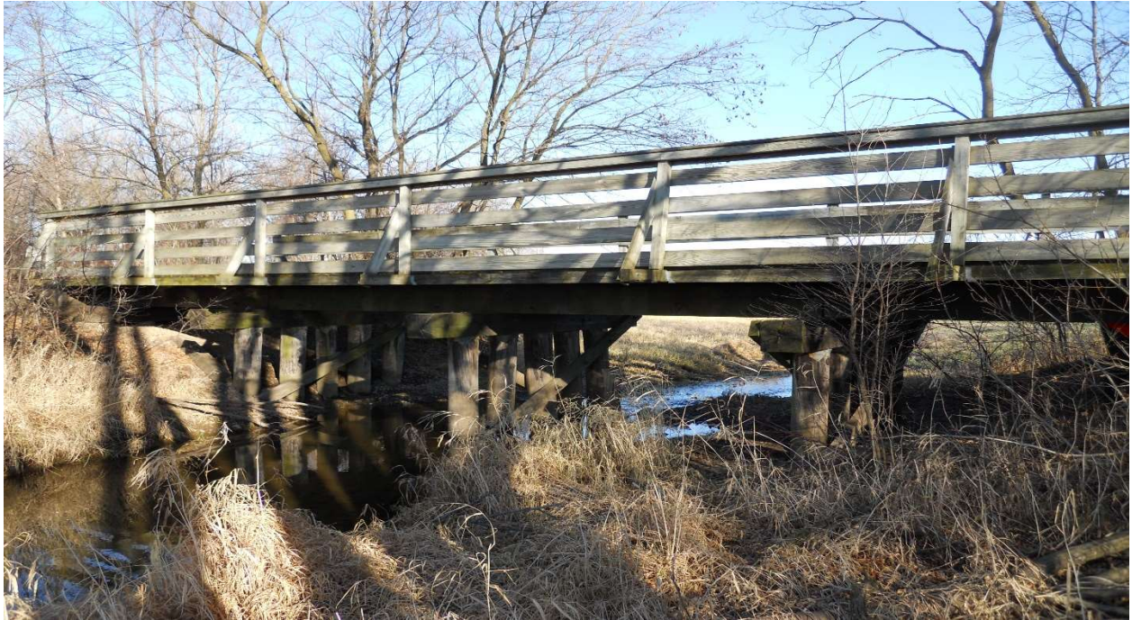
South fascia, looking northwest.
