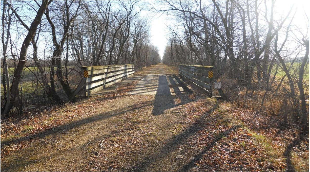
North approach, looking south.
