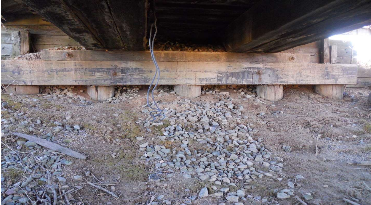
East abutment, looking east.
