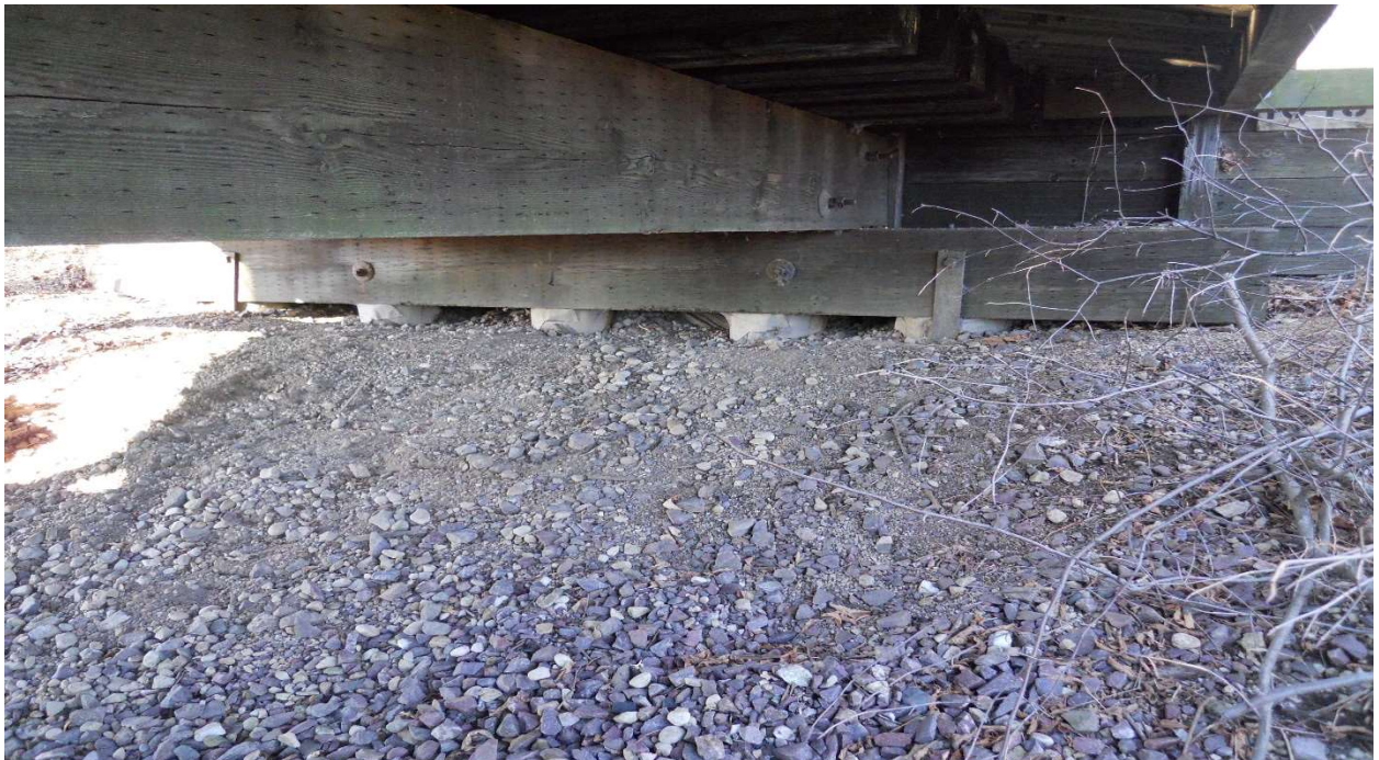
West abutment, looking southwest.
