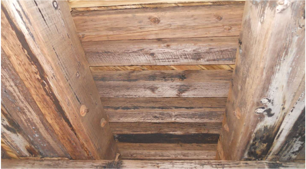
Underdeck, looking west.
