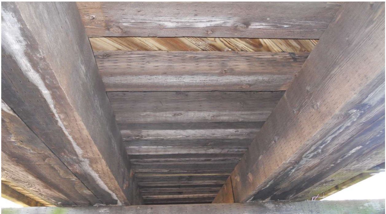
Underdeck, looking northwest.
