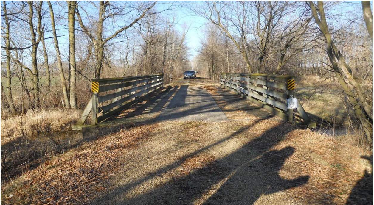
South approach, looking north.
