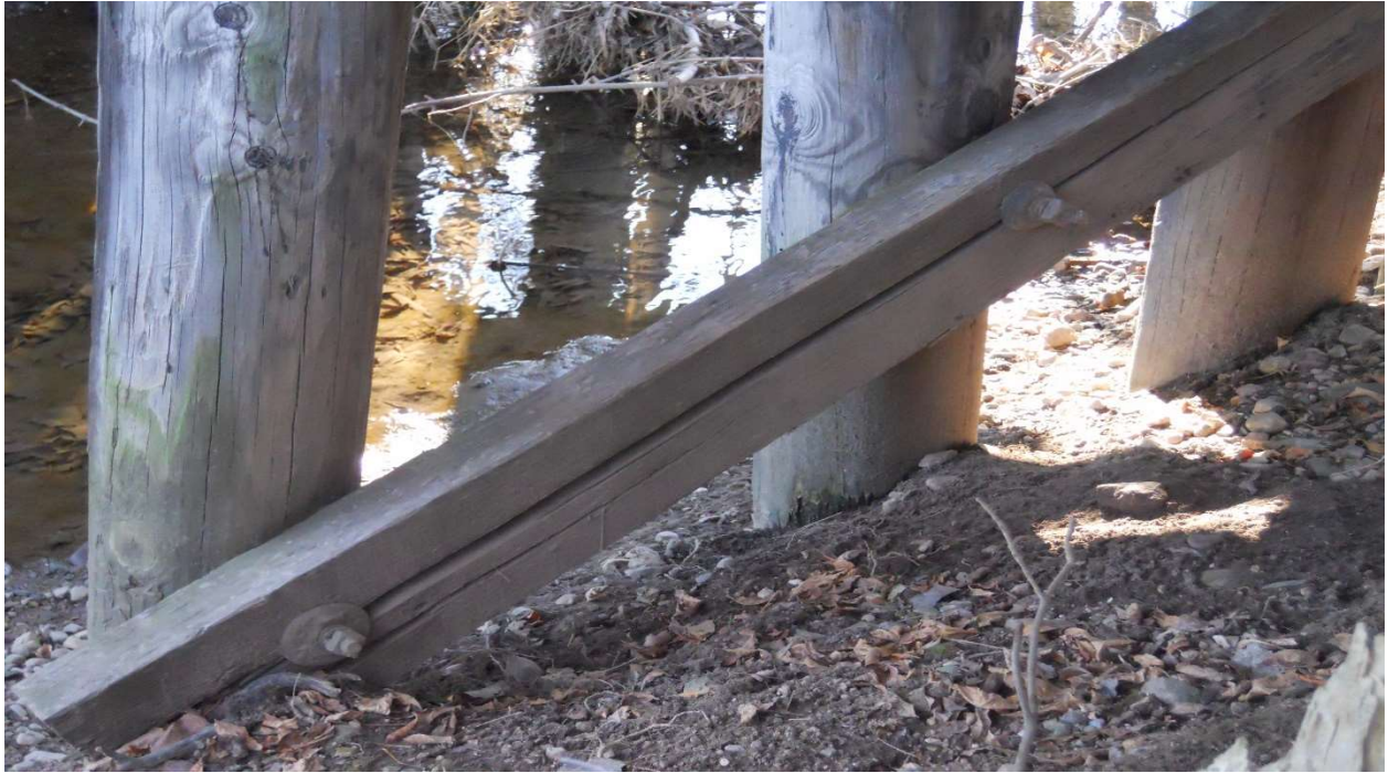
Split cross brace, west pier, looking south.
