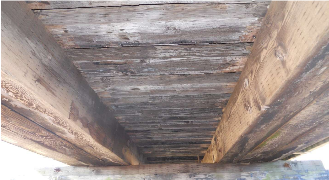
Underdeck, looking west.
