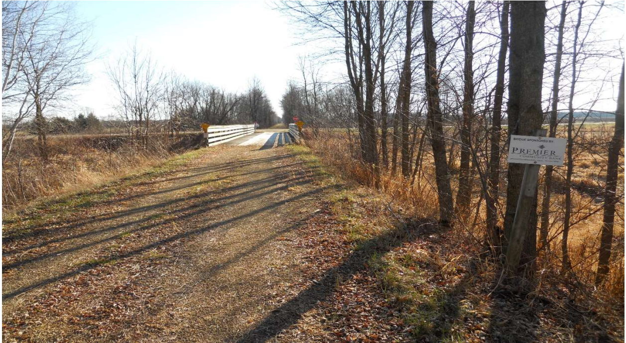
West approach, looking east.
