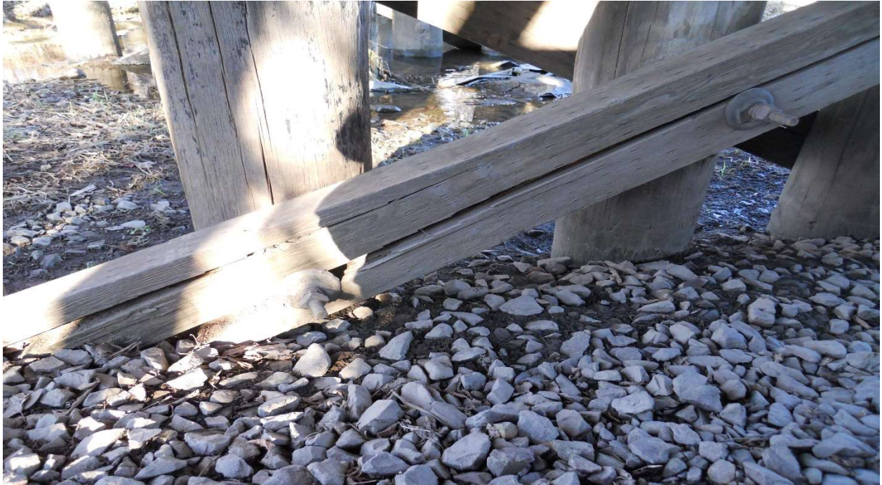
Split diagonal/cross brace, looking west.
