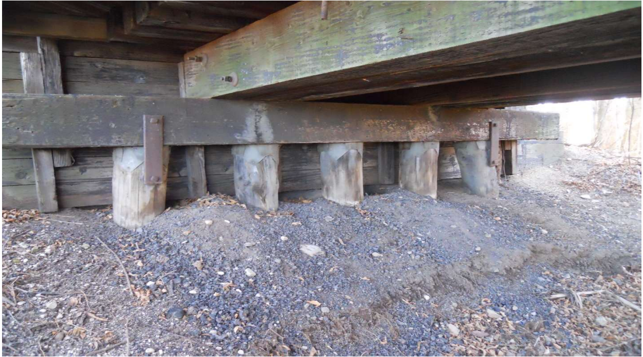
West abutment, looking southwest.
