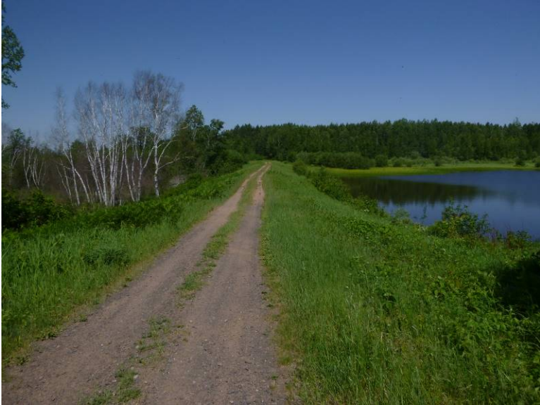
Embankment facing NW.
