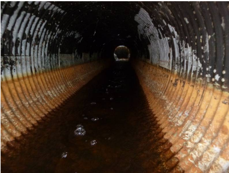
Interior of pipe.
