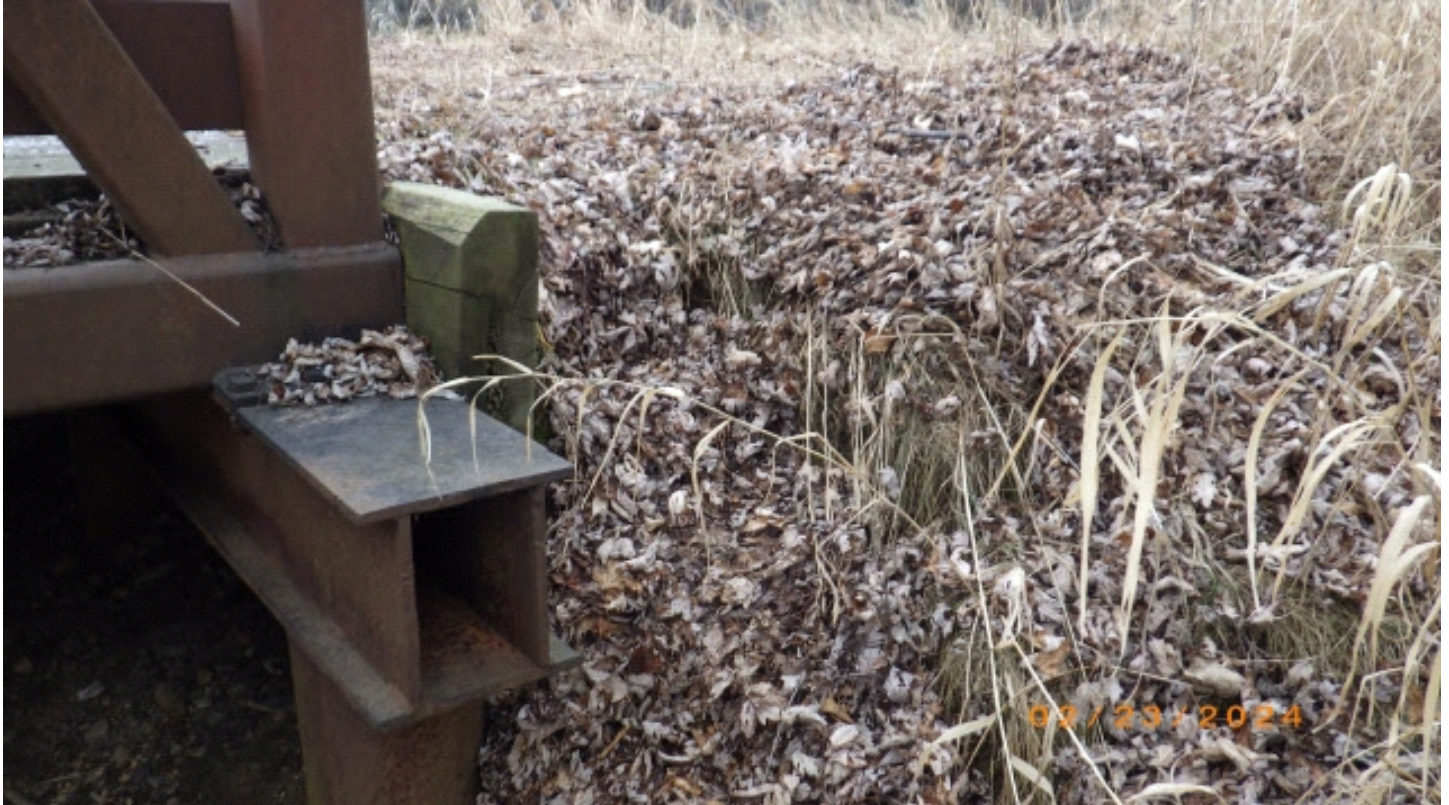
Fix erosion SE corner.
