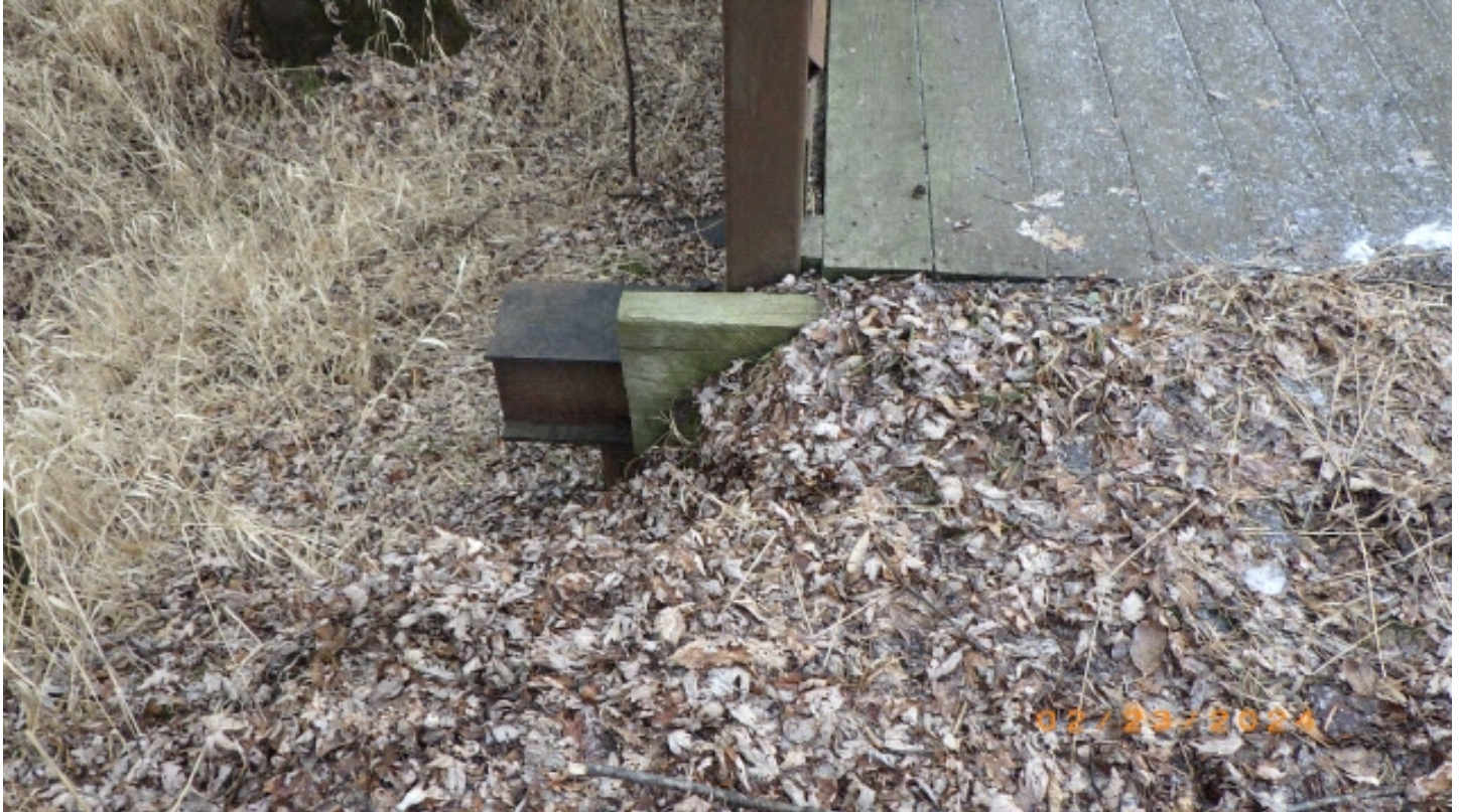
Fix Erosion NE corner.
