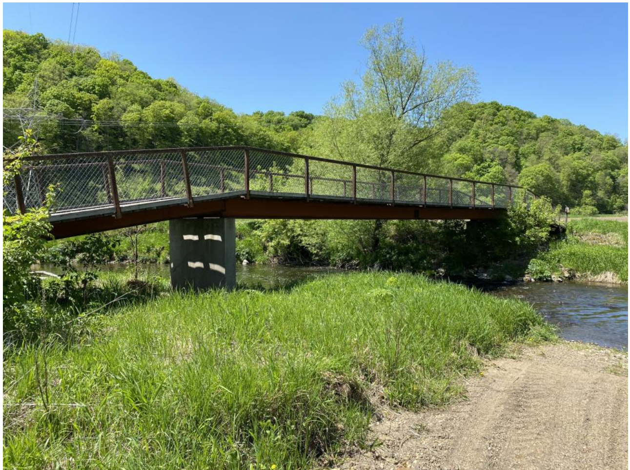
This may be because of the span over such narrow concrete supports
