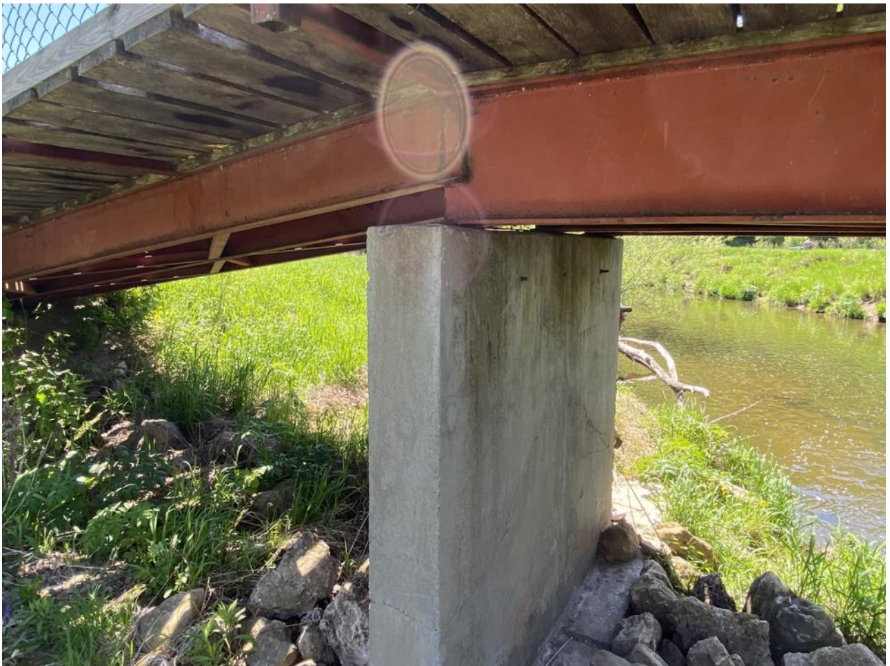
Set high on narrow concrete abutments. The main structure is also very narrow.
