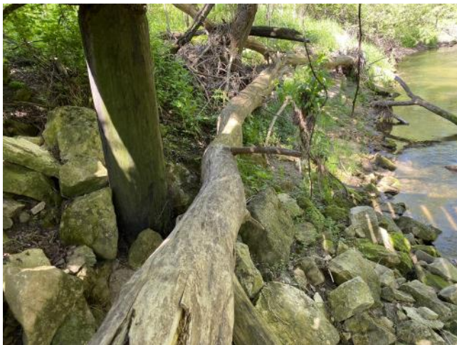
South end has some rip rap. Washed trees need to be removed.
