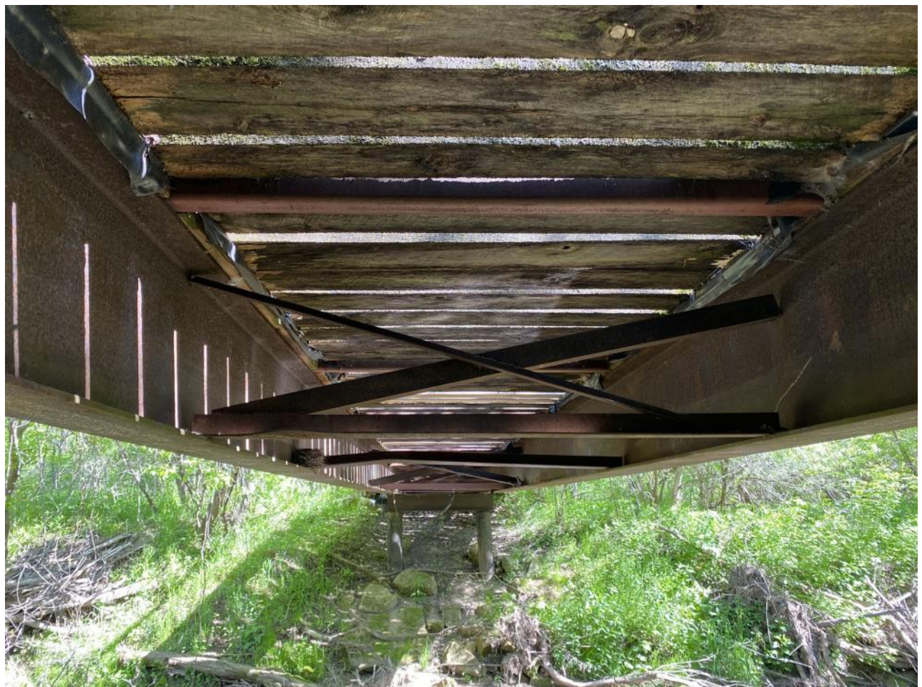
North end. Also showing cross members and deck condition
