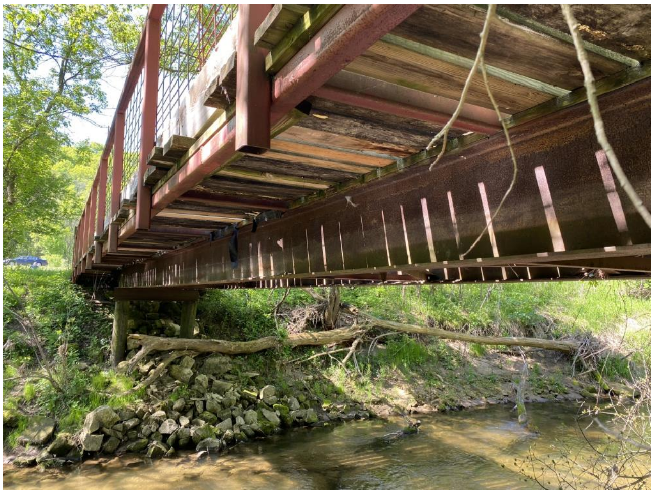
South end has some rip rap. Washed trees need to be removed.
