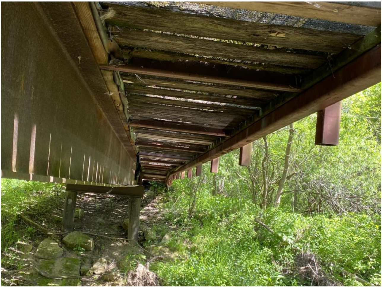
This is what is supporting the groomers. Wooden decking and
