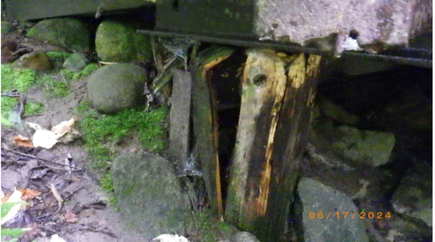
Extra support of Failed West Pier.
