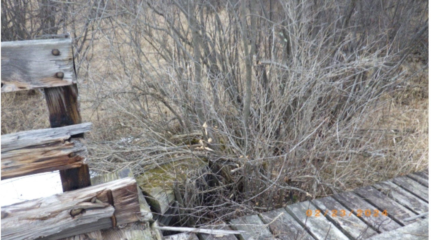
Damaged Railing
