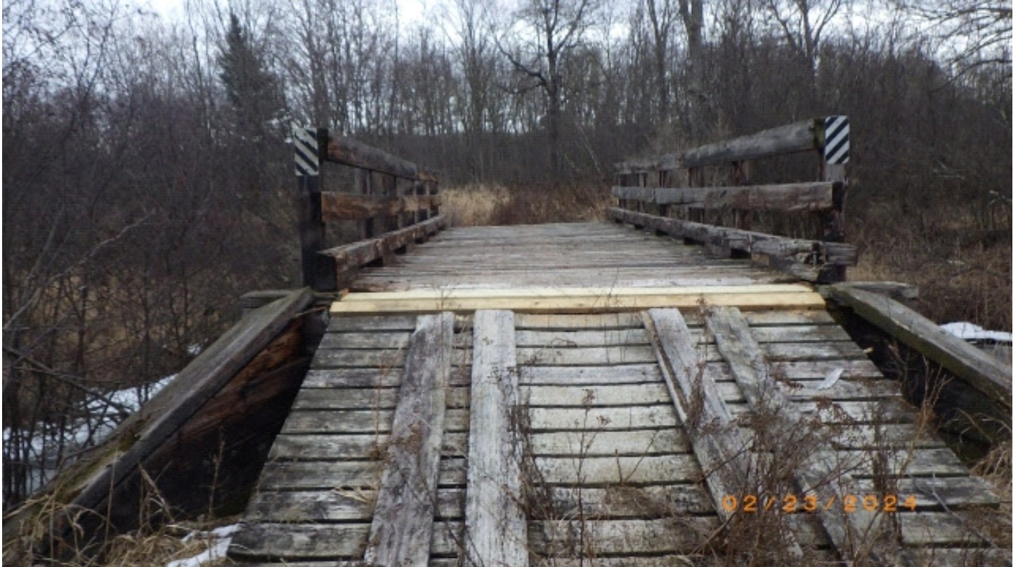
Approach and few replaced boards.
