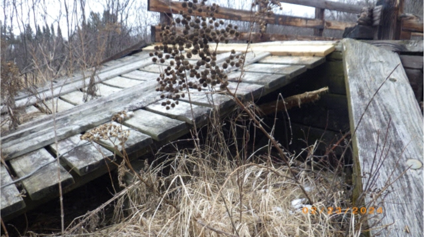
West approach span
