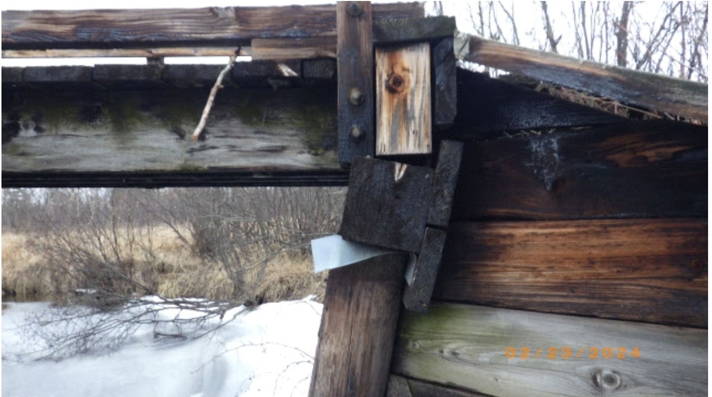
Rotating pile cap.
