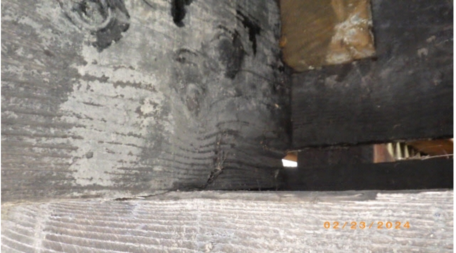
Crushing girders and approach span sitting on backing boards.
