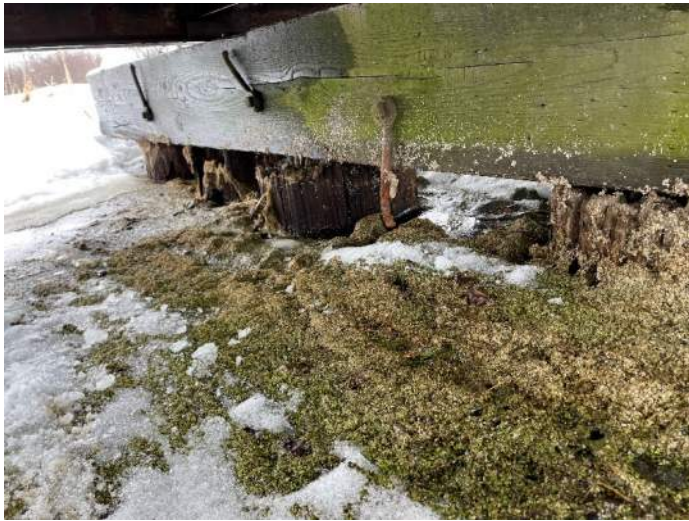
Typical pile condition at pier
