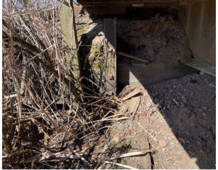
Typical Timber abutment (E)
