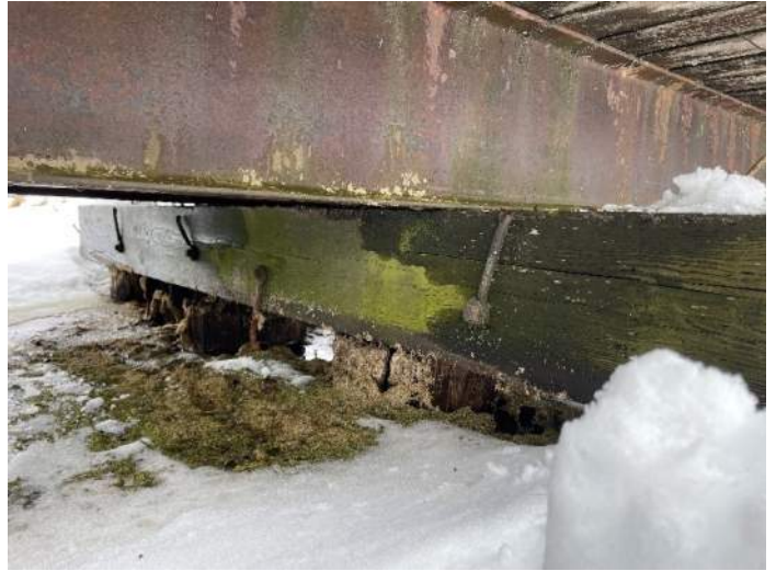
Typical bearing at pier
