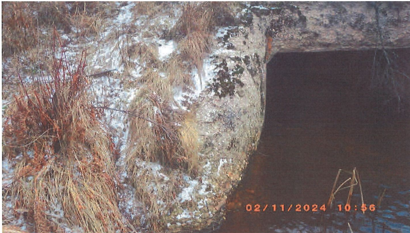
NW wingwall section loss
