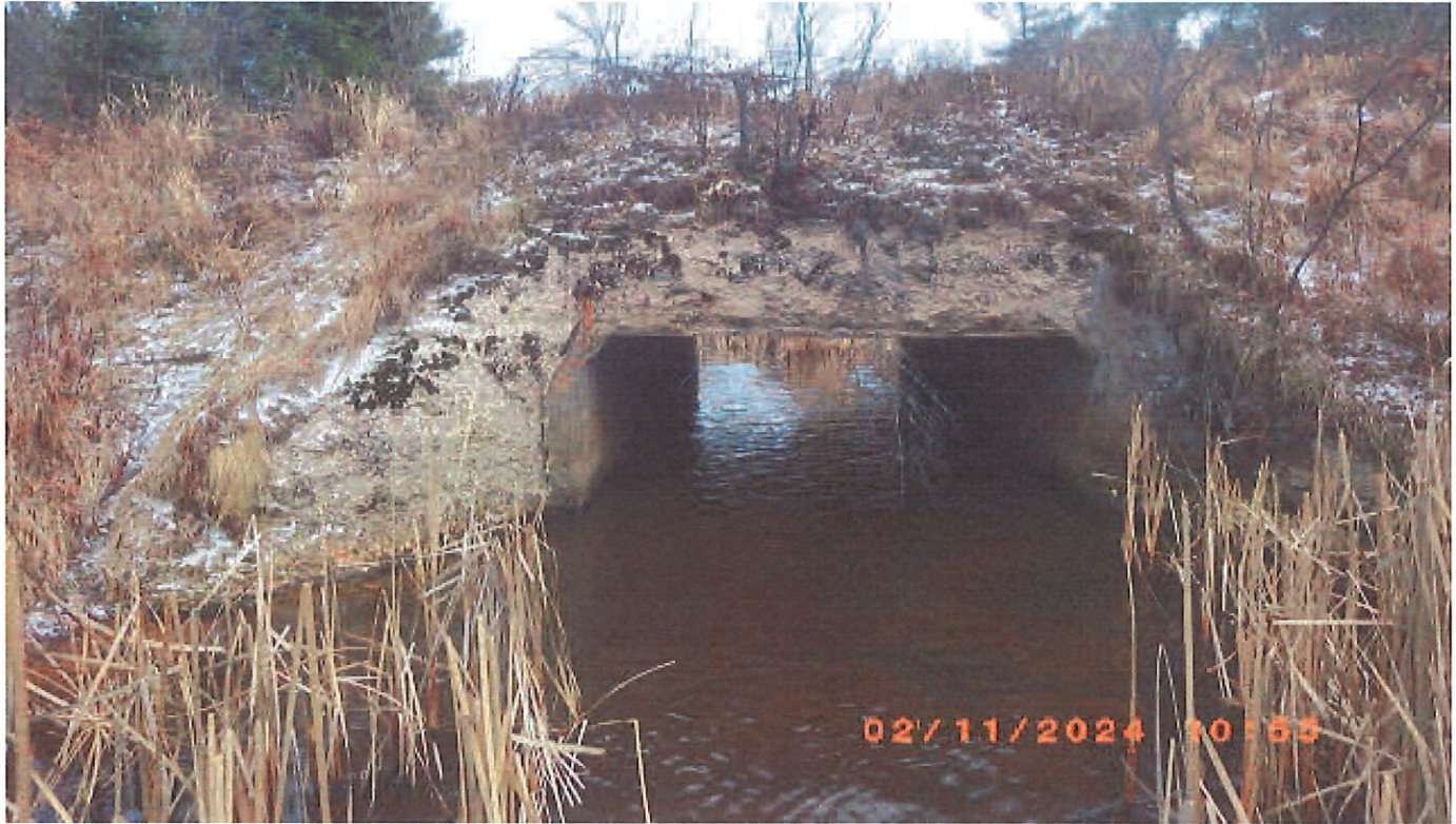
Outlet elevation view
