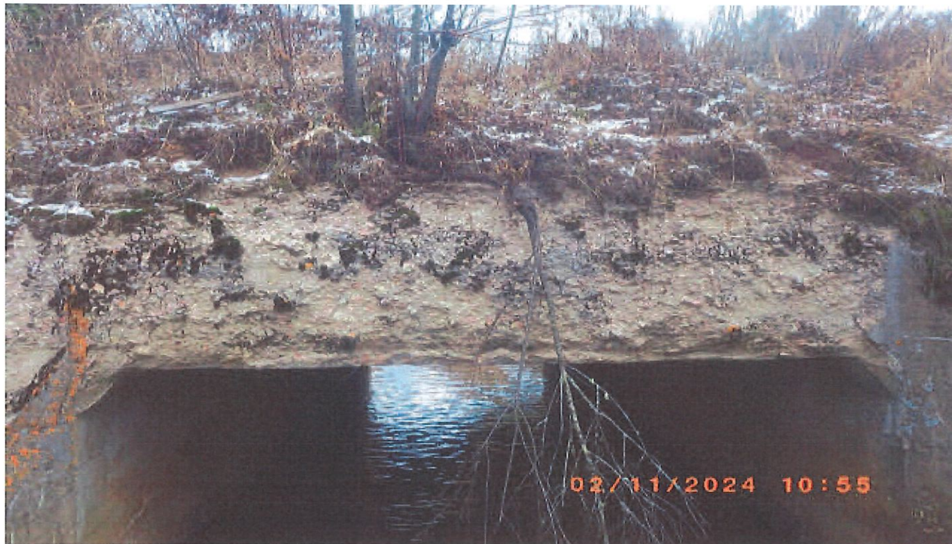
Top of box / headwall, west side
