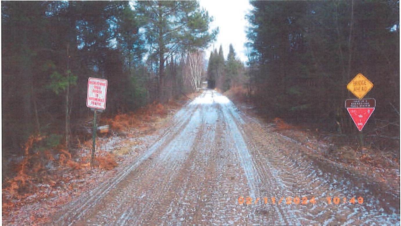
South bridge ahead / other signs
