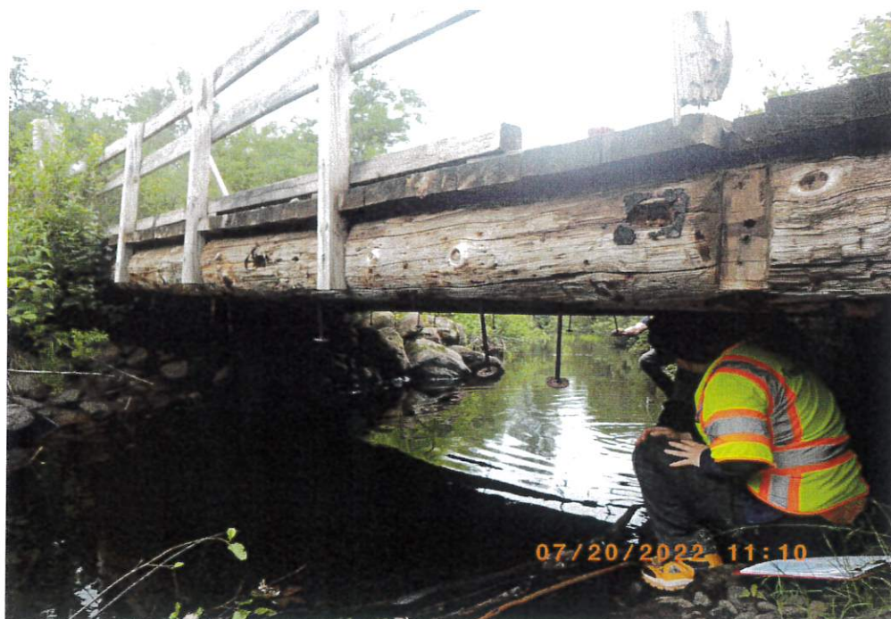
Looking Downstream - Elevation Profile
