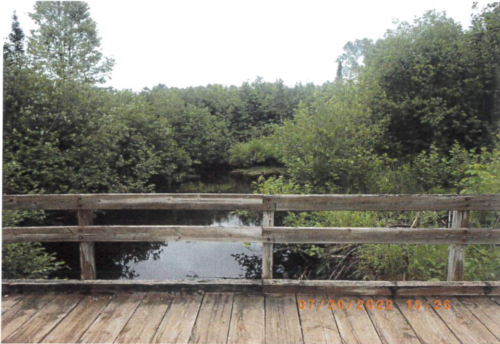
Looking Upstream from the Bridge Deck
