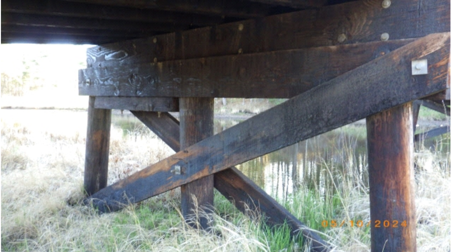
Pier along channel, typical.
