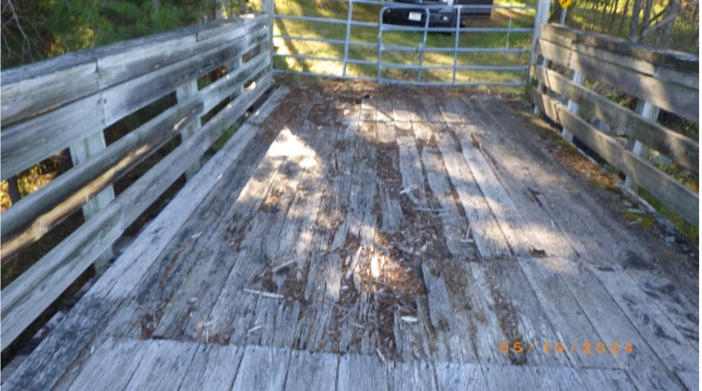
CS4 wearing surface, typical.
