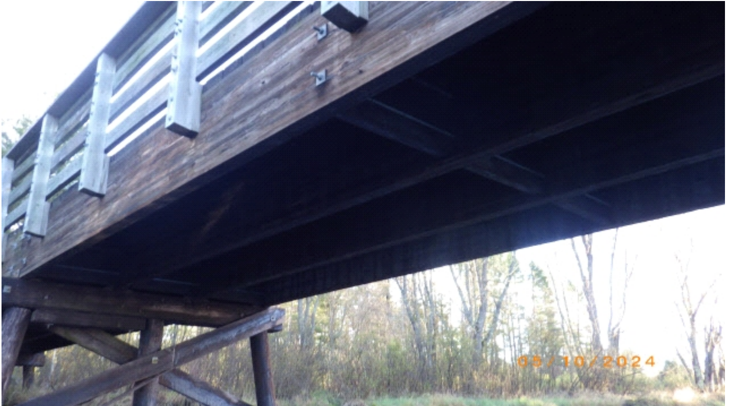
Glulam Span, typical.
