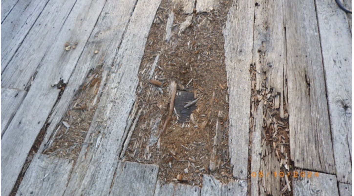
CS4 Wearing surface, typical.
