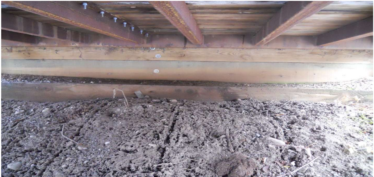
North abutment, looking north.
