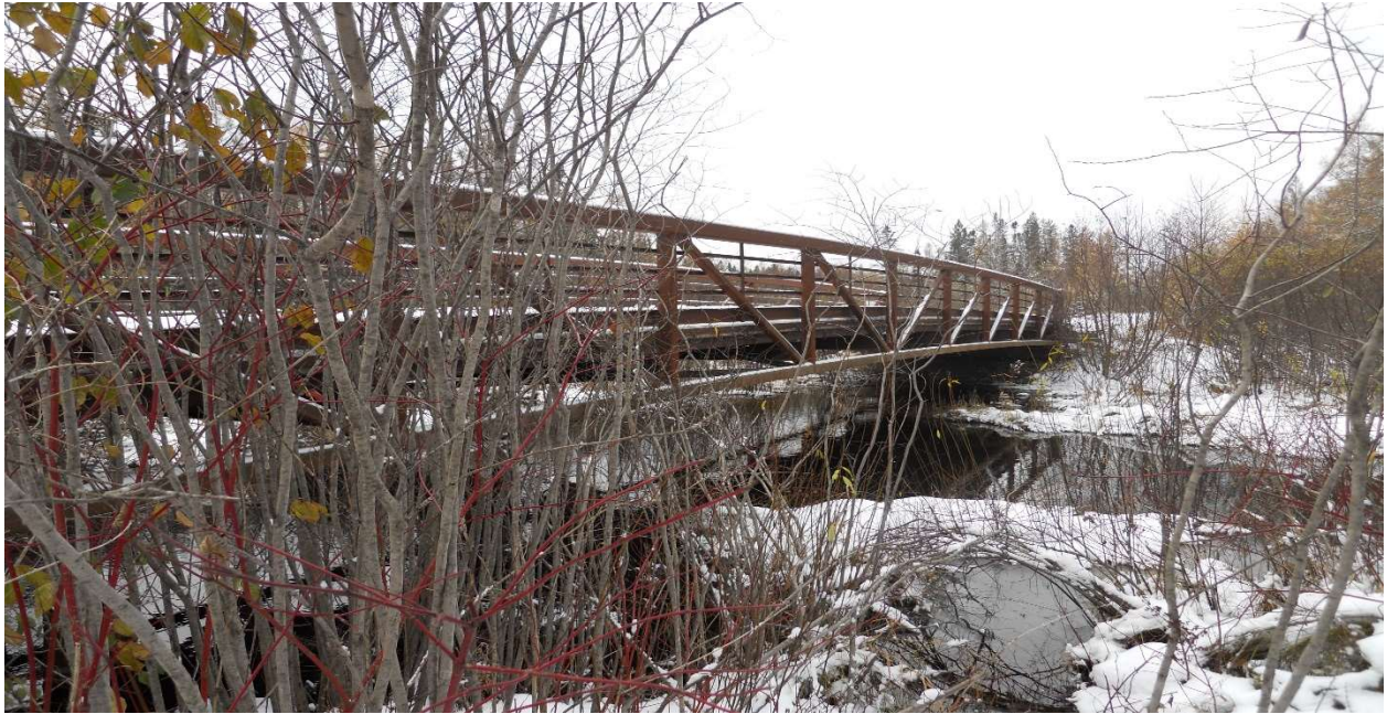
West fascia, looking southeast.
