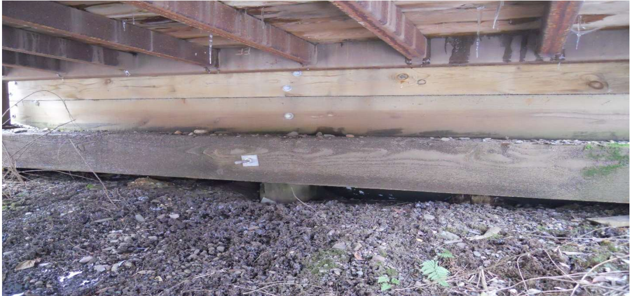
South abutment, looking south.
