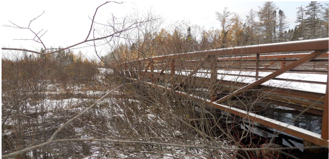
East fascia, looking southwest.
