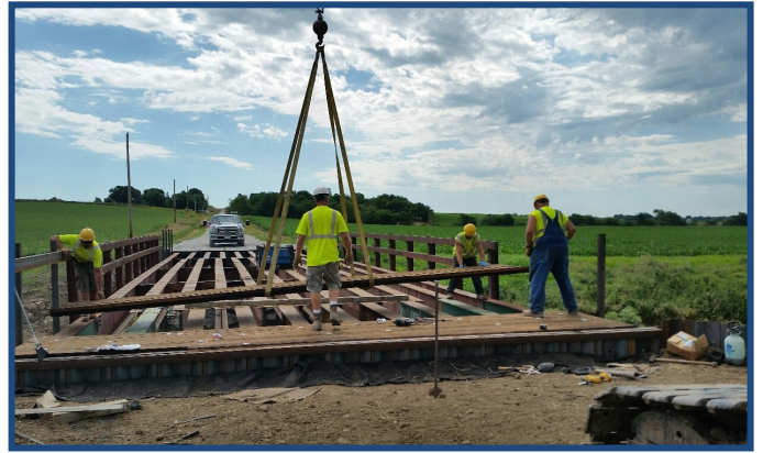
Handled w/ Small Crane
