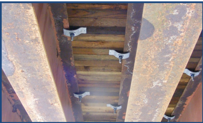
Finished Panel/Stringer Connection
