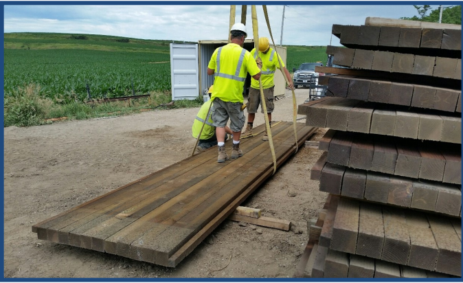
New Timber Deck Panels
