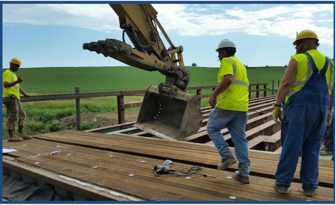
Panels Set on Steel Stringers
