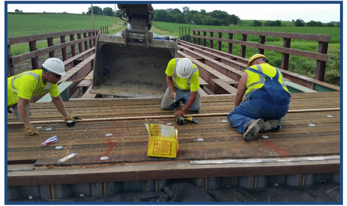
Panels Interconnect via Ship-lap
