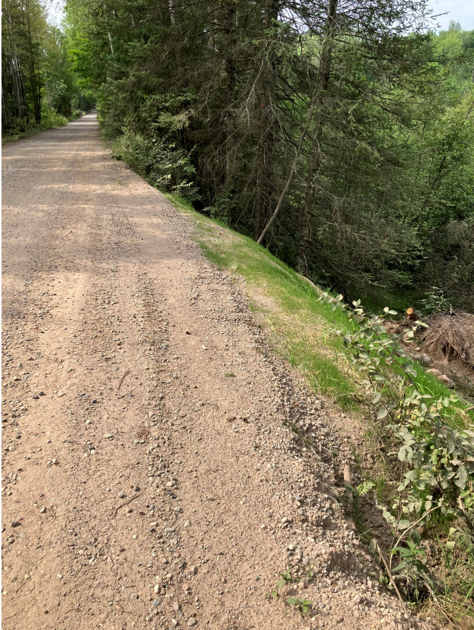
Forest County, Nicolet Trail Storm Damage – AFTER repairs
