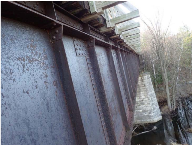
Main steel plate girders
