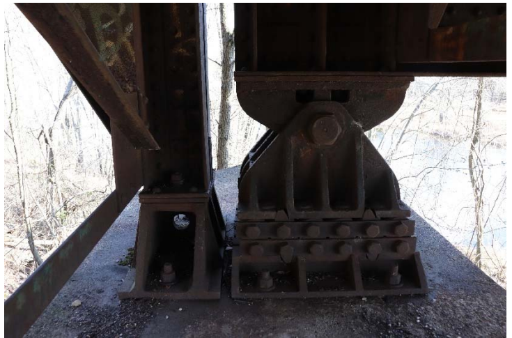
Cracked bearing at pier 3, east side
