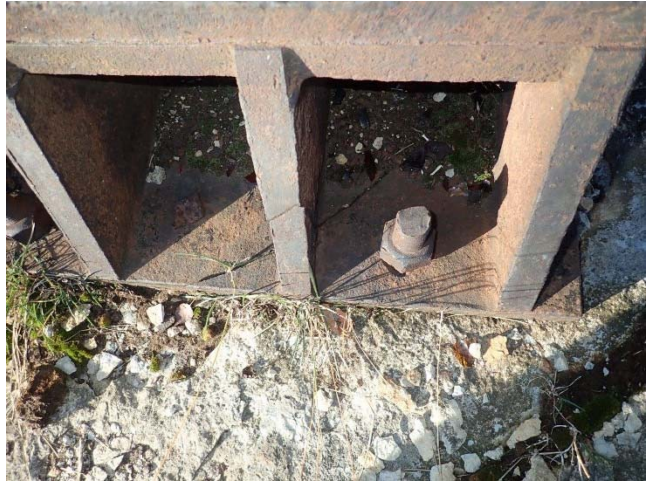
Cracked bearing at pier 3, east side
