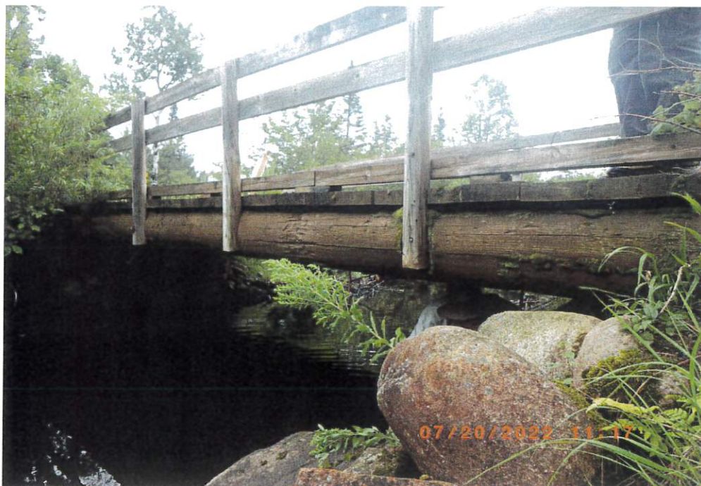
Looking Upstream - Elevation Profile
