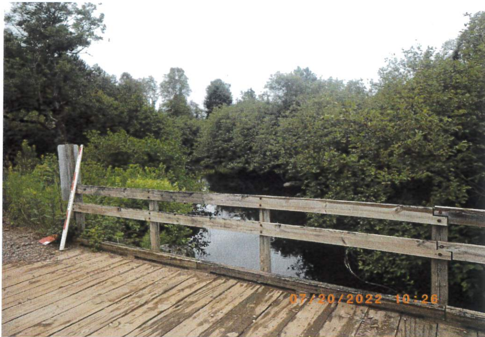
Looking Downstream from the Bridge Deck
