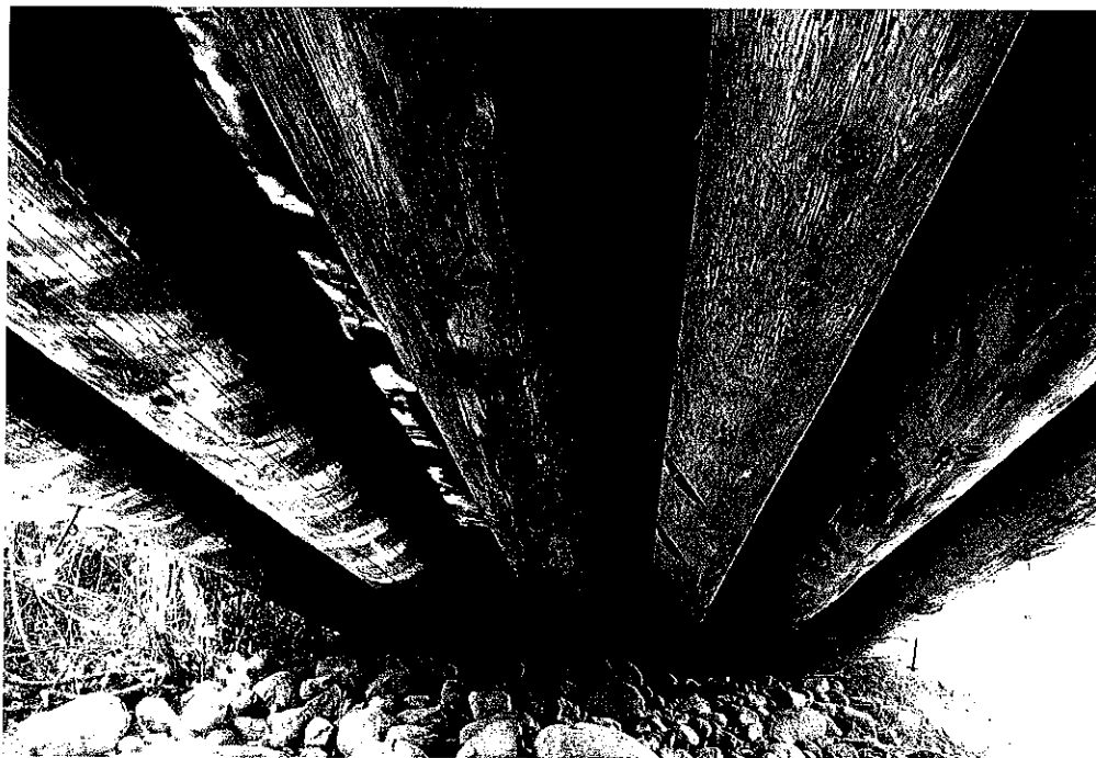
View of Superstructure
