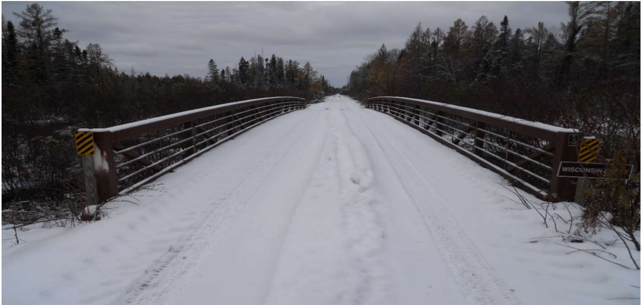
North approach, looking south.
