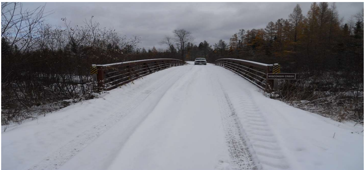
South approach, looking north.
