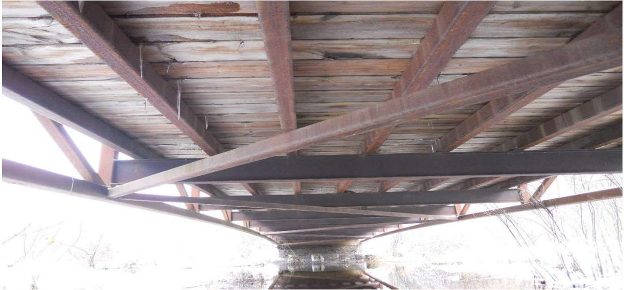
Underdeck, looking north.
