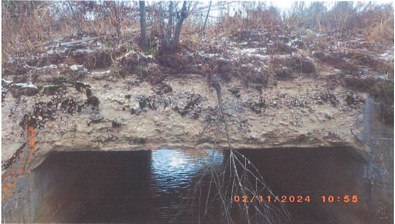
Top of box / headwall, west side
