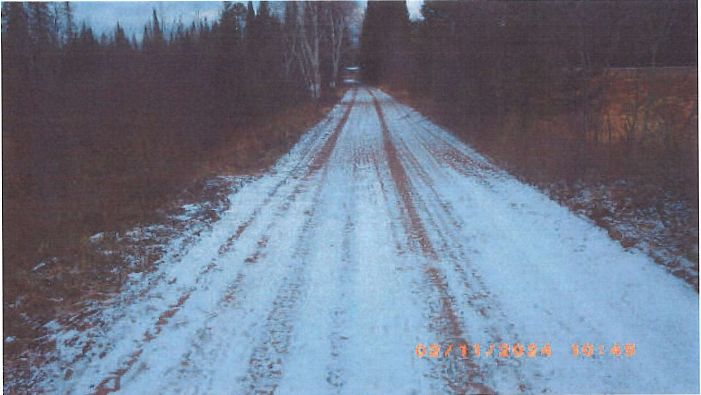
CS3 Roadway over structure
