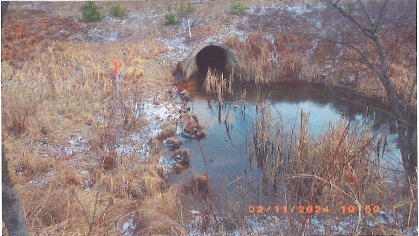
Looking upstream (highway culvert)
