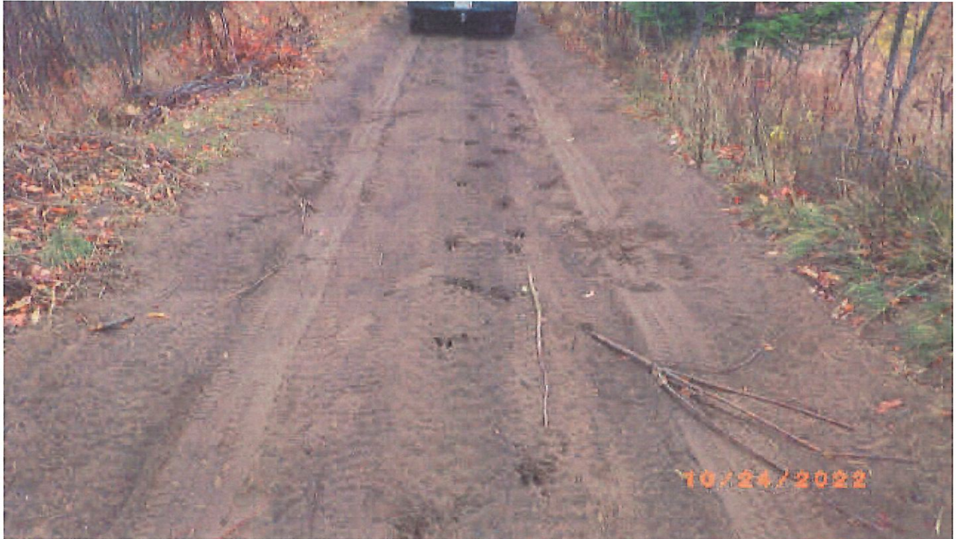
2022 CS3 road way over structure.
