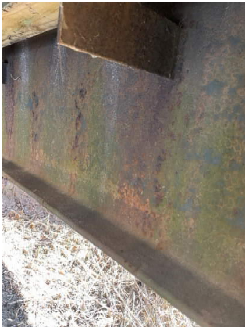
Typical Girder condition
