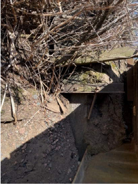
Typical Timber abutment (E)
