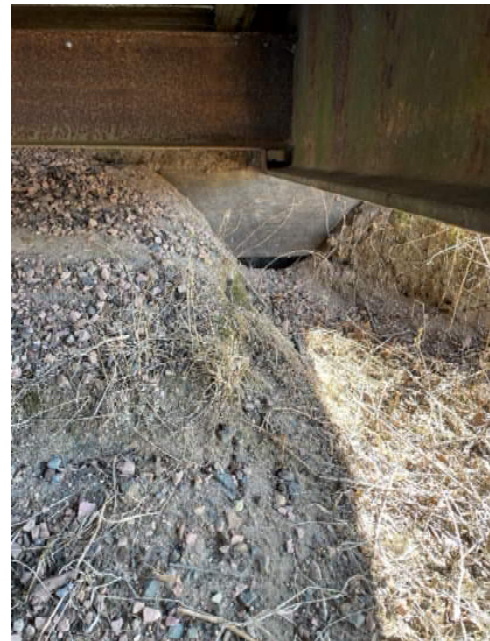
Typical Timber abutment (W)
