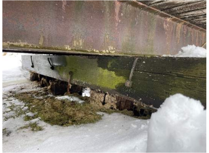
Typical bearing at pier
