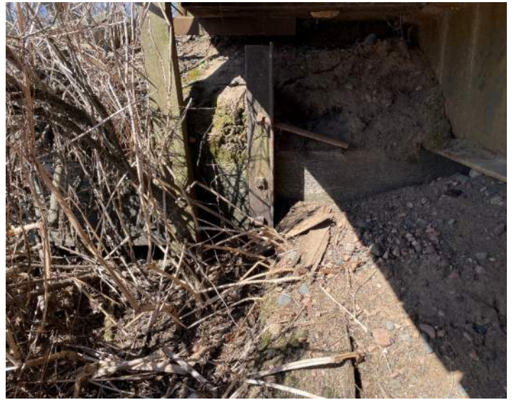
Typical Timber abutment (E)
