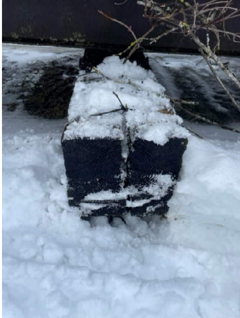
Typical timber pier cap
